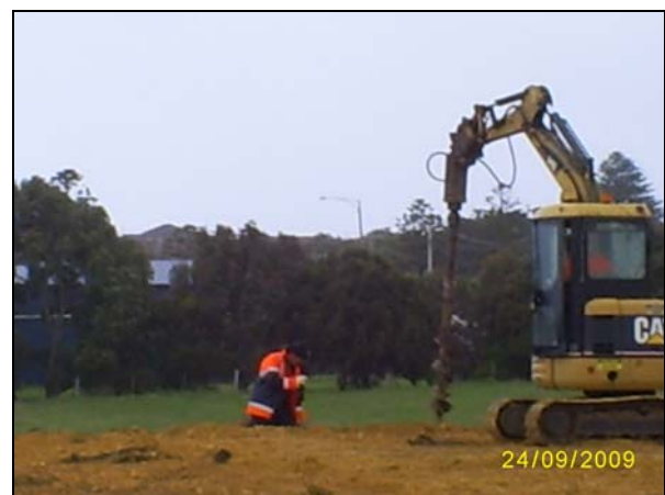
Drilling the piers
