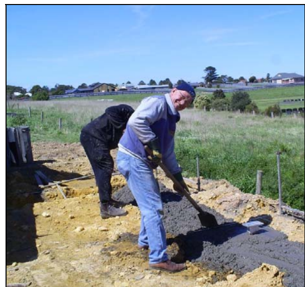
"Happy Shedder", Peter Fawns helps in pouring beams
