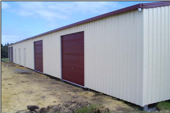
The Shed – erected at last!
