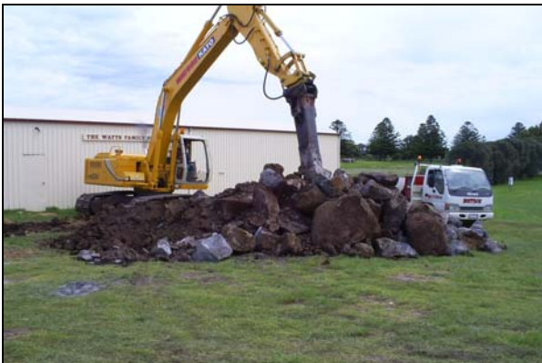
A lot of rock came out for the tank!
