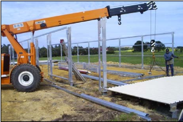
Raising the end walls
