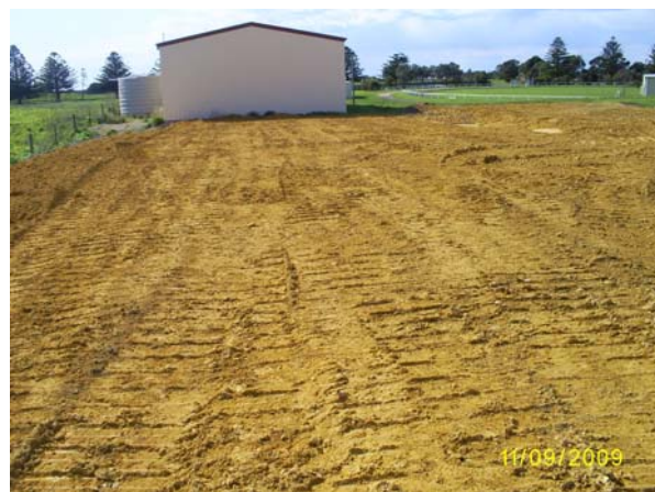
The Shed site ready for construction
